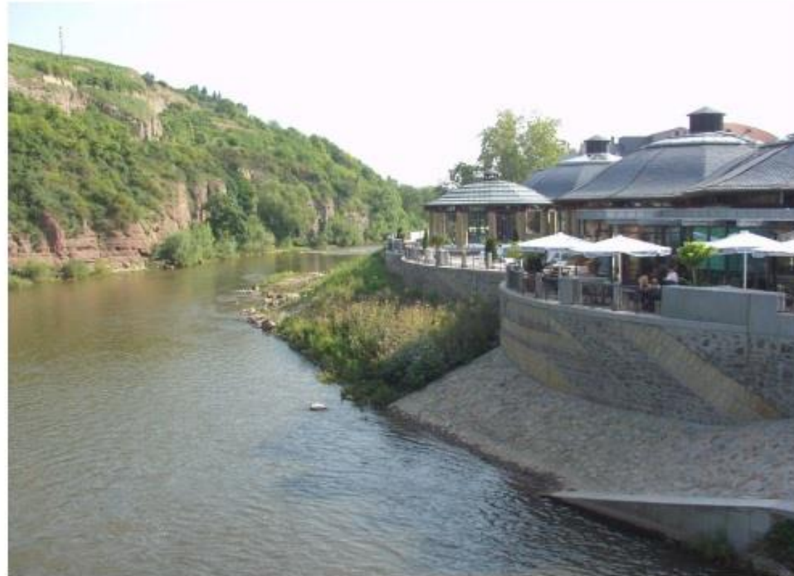
Flood protection Bad Kreuznach
