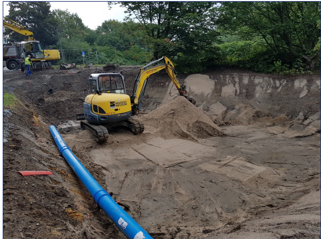
Abb. 19: RRB A = \text{ca. } 145 \text{ m}^2 , V = \text{ca. } 65 \text{ m}^3
